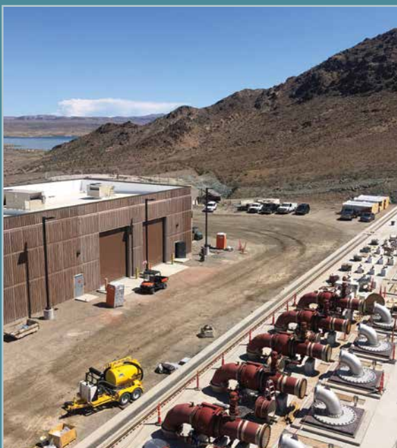
Low Lake Level Pumping Station Construction
