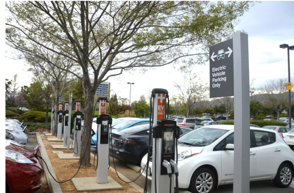
EV charging station installation.
